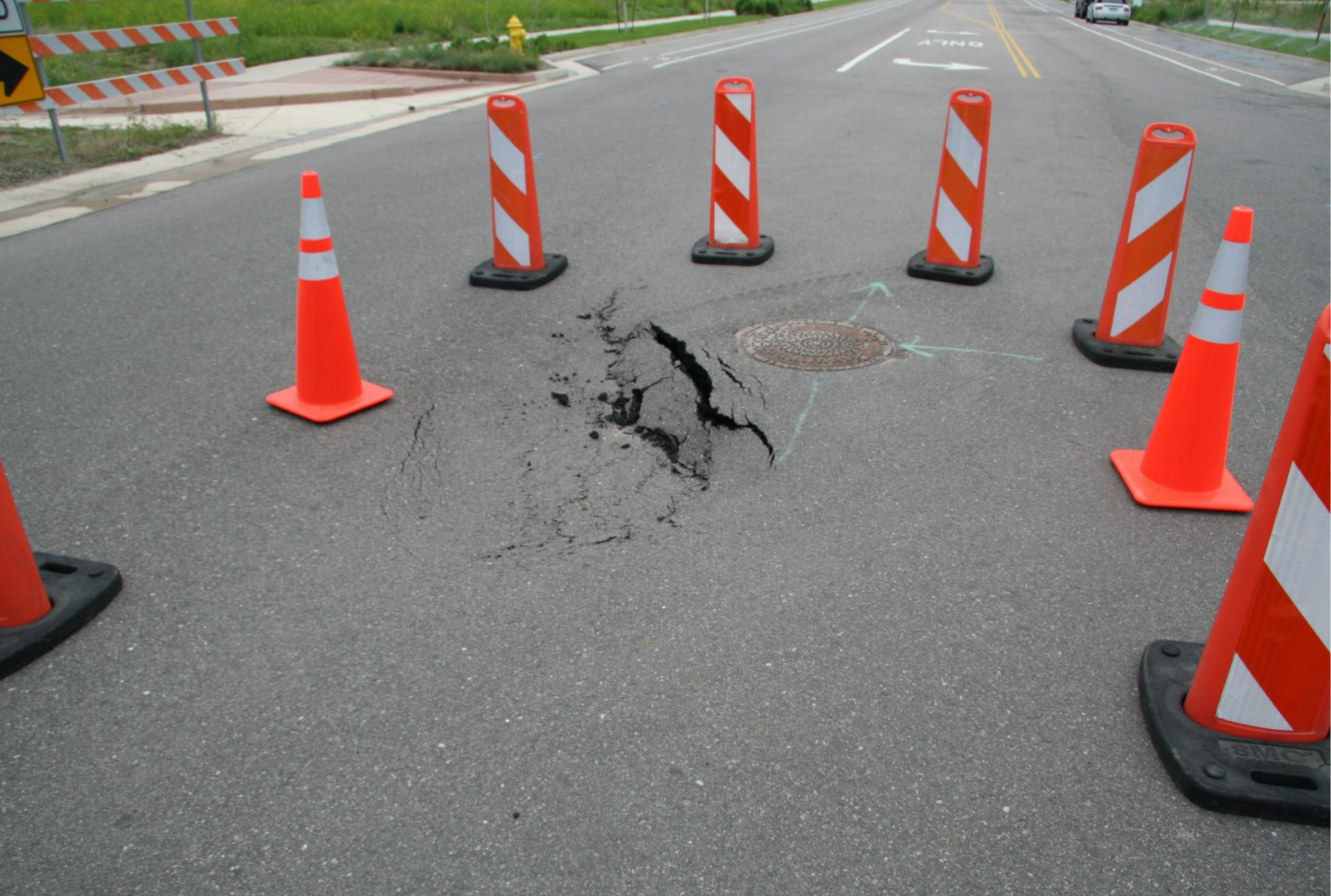
Photo 1 June 4, 2009 Project No. DN 43,846-145
