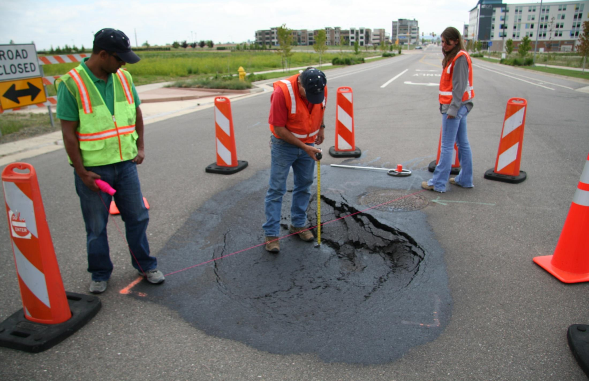
Photo 355 June 8, 2009 Project No. DN 43,846-145
