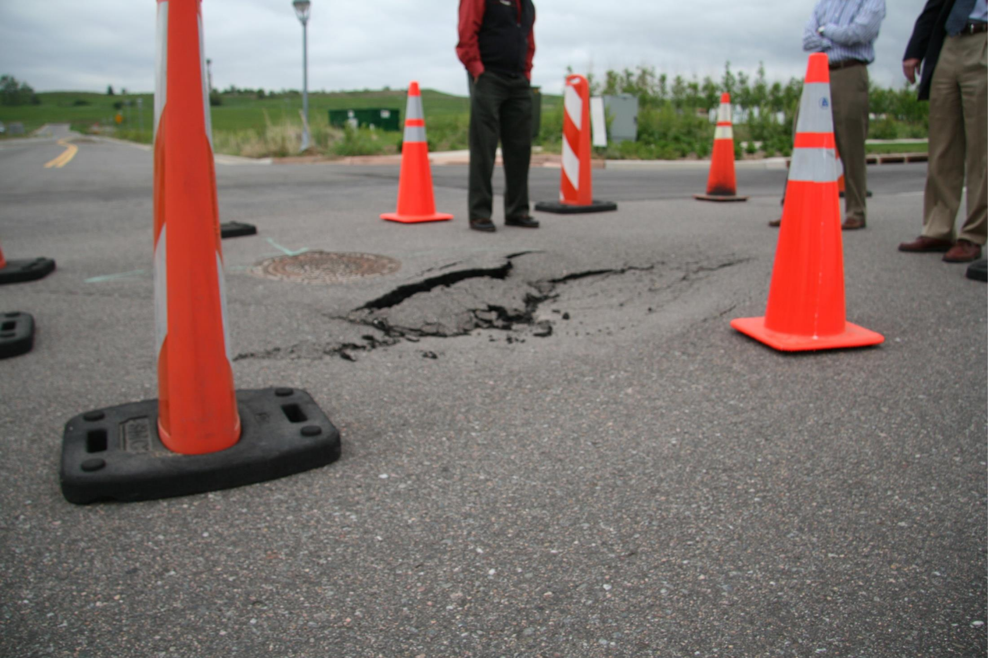
Photo 2 June 4, 2009 Project No. DN 43,846-145
