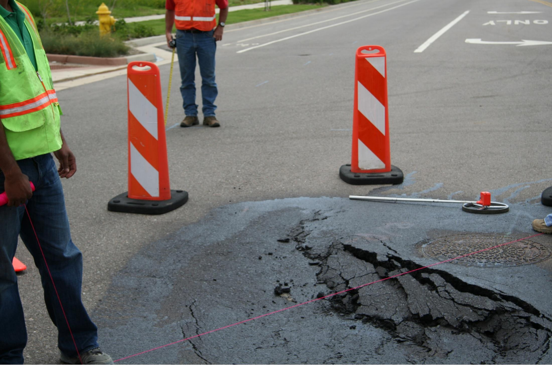
Photo 358 June 8, 2009 Project No. DN 43,846-145
