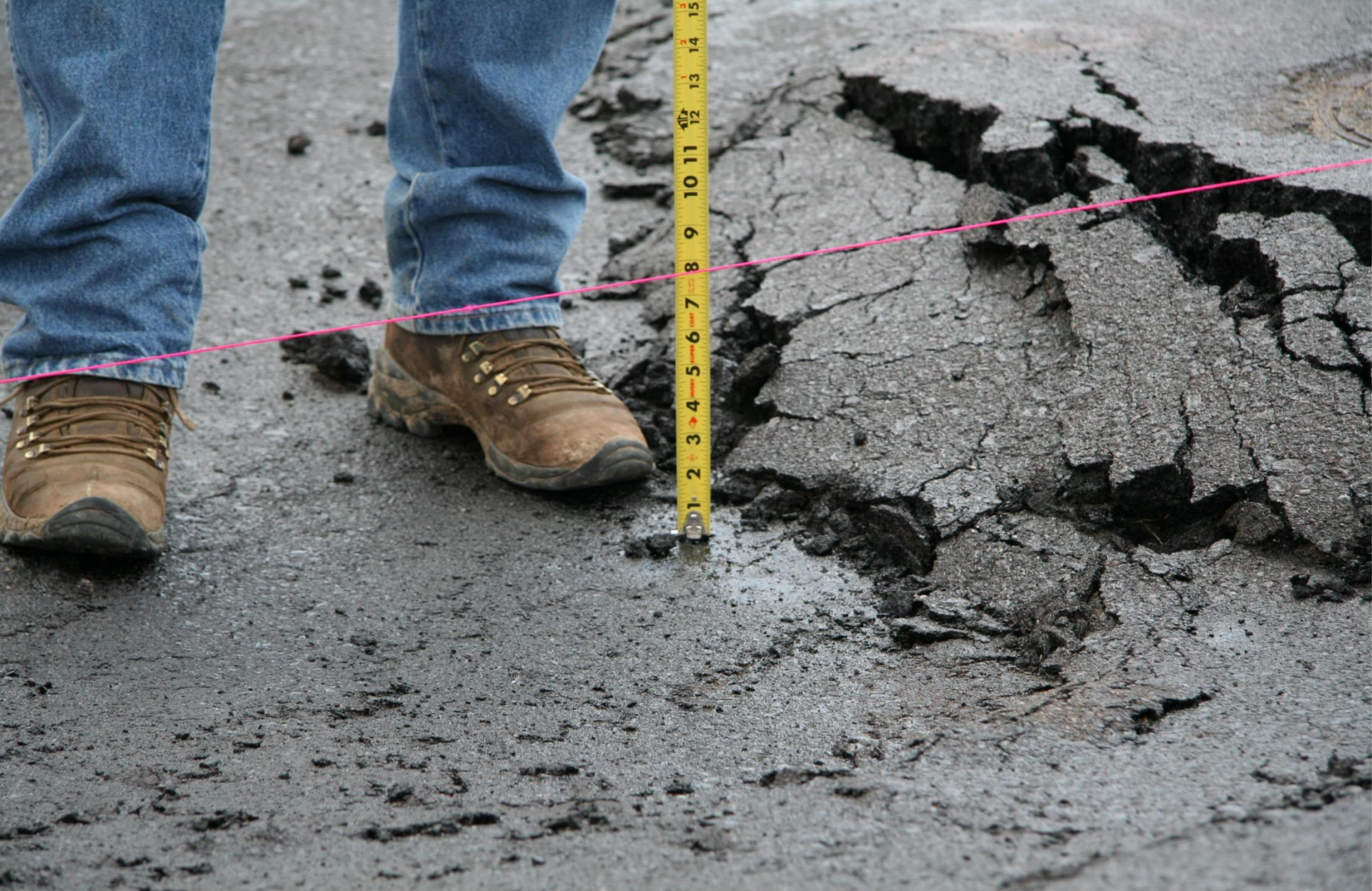
Photo 356 June 8, 2009 Project No. DN 43,846-145
