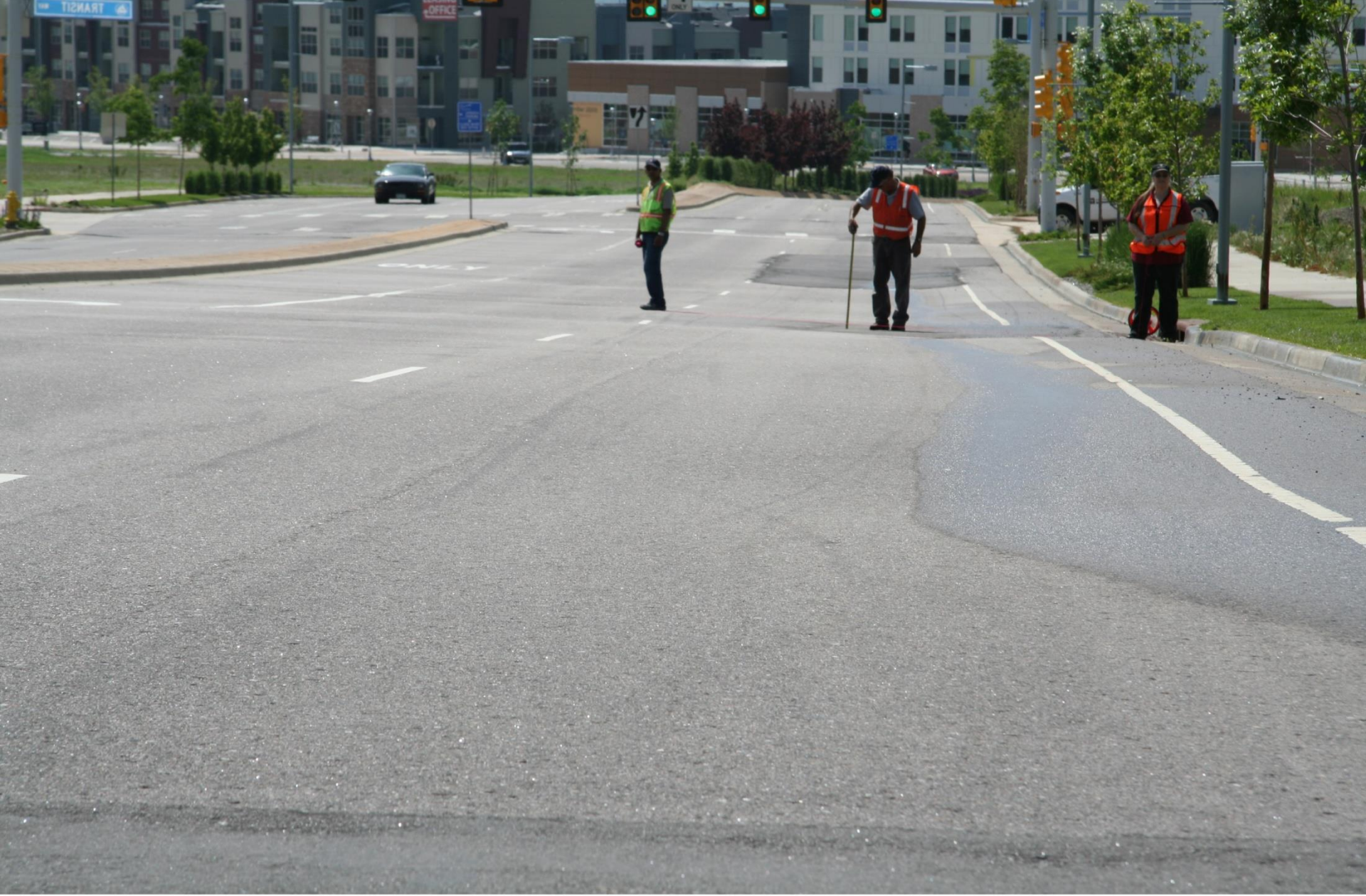
Photo 81 June 5, 2009 Project No. DN 43,846-145
