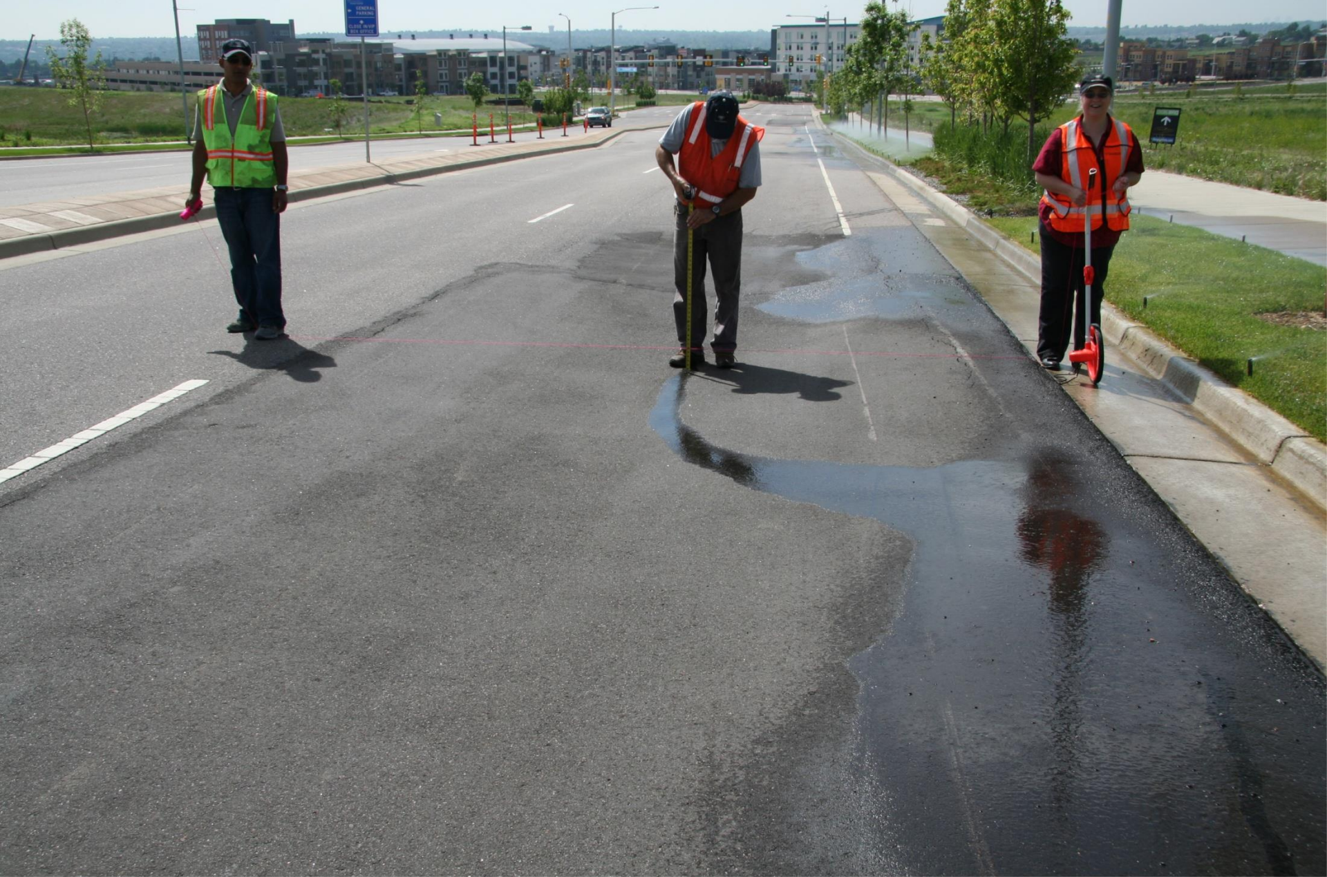
Photo 63 June 5, 2009 Project No. DN 43,846-145
