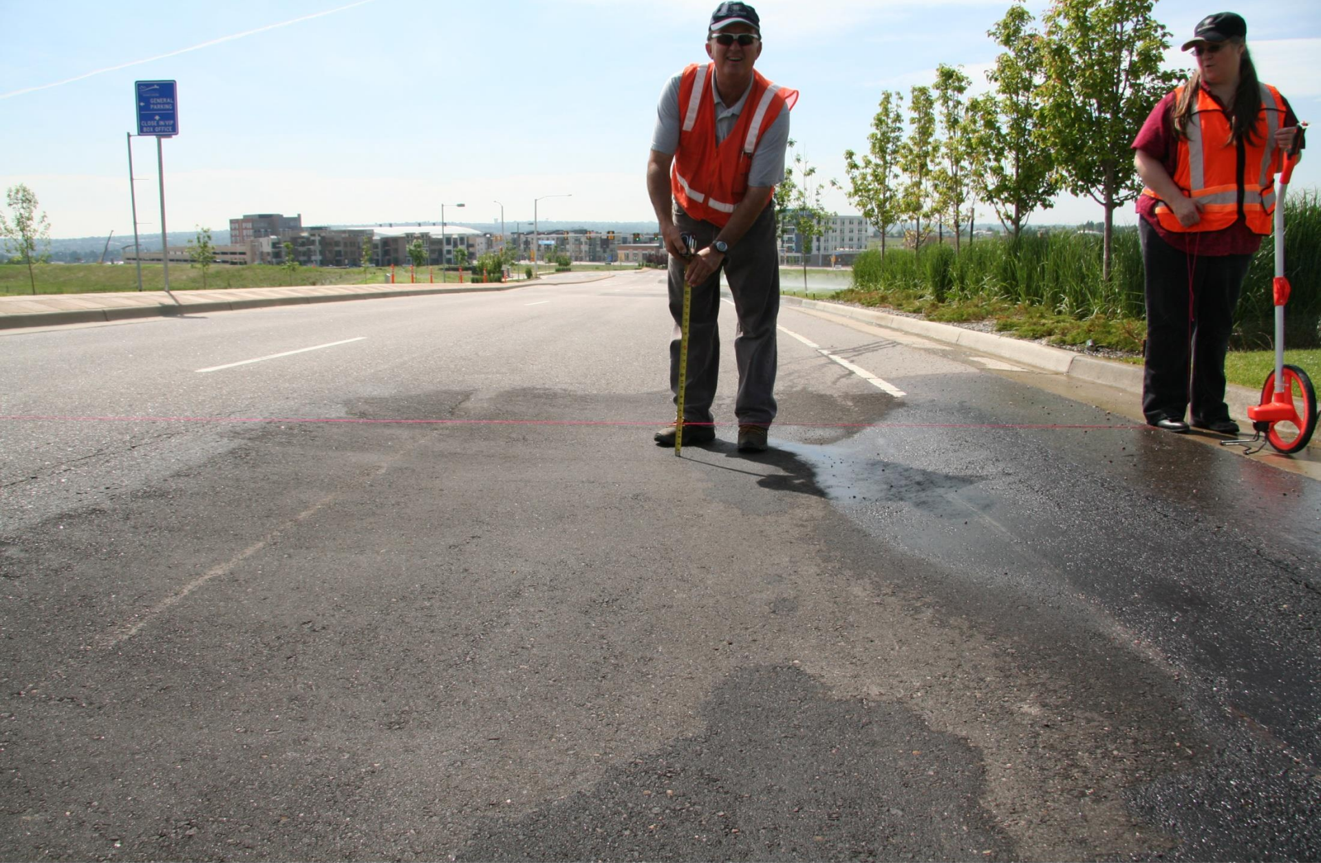
Photo 66 June 5, 2009 Project No. DN 43,846-145
